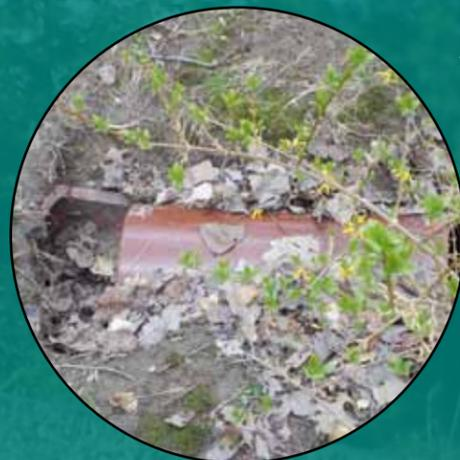
Repair or replace visible shallow broken pipes to prevent storm water from infiltrating your sewer system and eliminate the chance of clogging.
