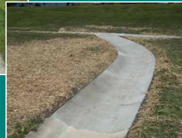
Replaced concrete channel at Fire Station #3
