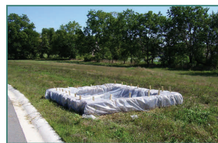
Hay bale and plastic washout pit
