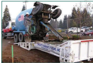
Metal washout container
