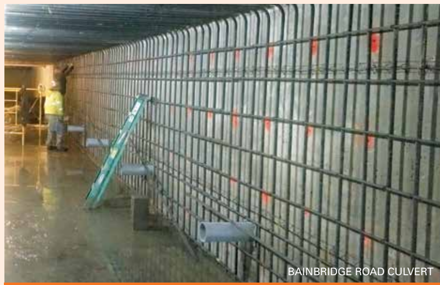
Lining of the box culvert under Bainbridge Road at Harper Road. Thank you for your patience with the road closure above this project.
