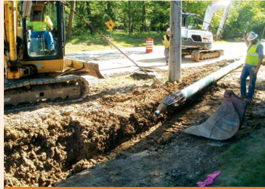
Pipe bursting 1,373 feet of sanitary sewer on Miles Road
